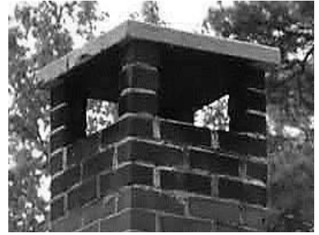
Concrete Cap Chimney Top
